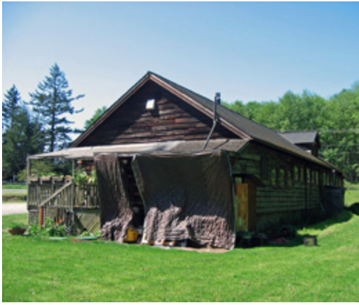
Strawberry Barreling Plant building, Olga, Orcas Island, 2006
