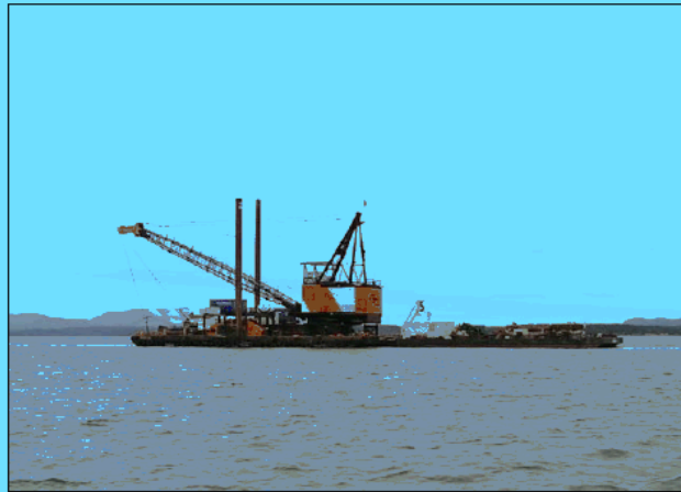
Figure 7 - Cable Repair Barge
