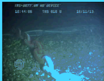
Figure 9 - Anchor Chain on Splice Box
